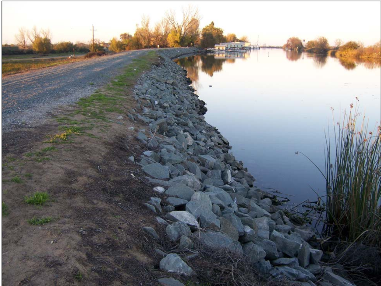
Figure 5-2: RD 799 Dutch Slough Levee
