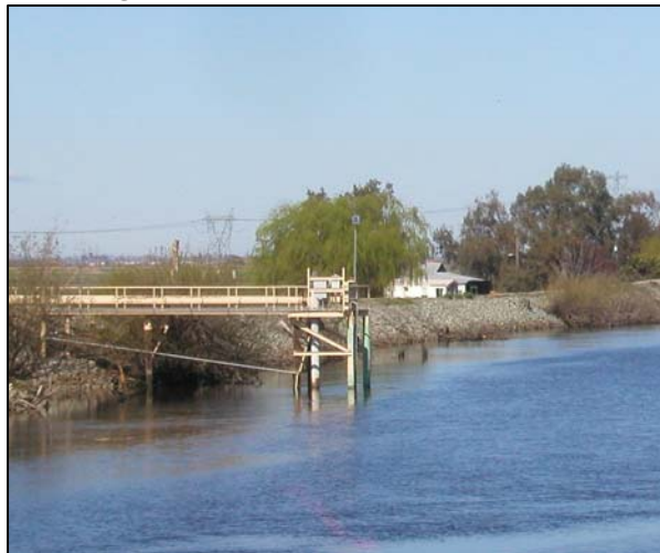
Figure 14-2: RD 2117 Old River Levee
