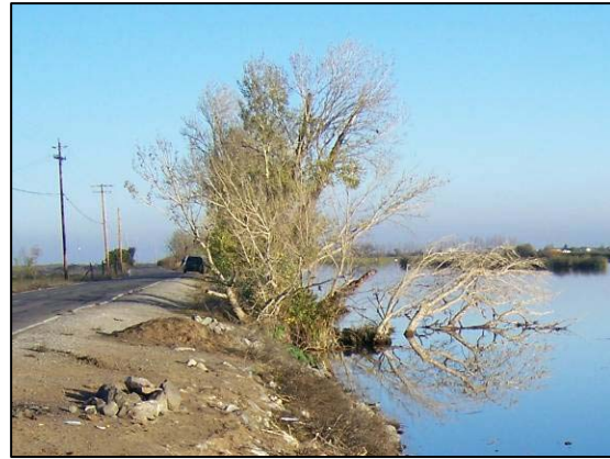
Figure 9-2: RD 2025 Rock Slough Levee
