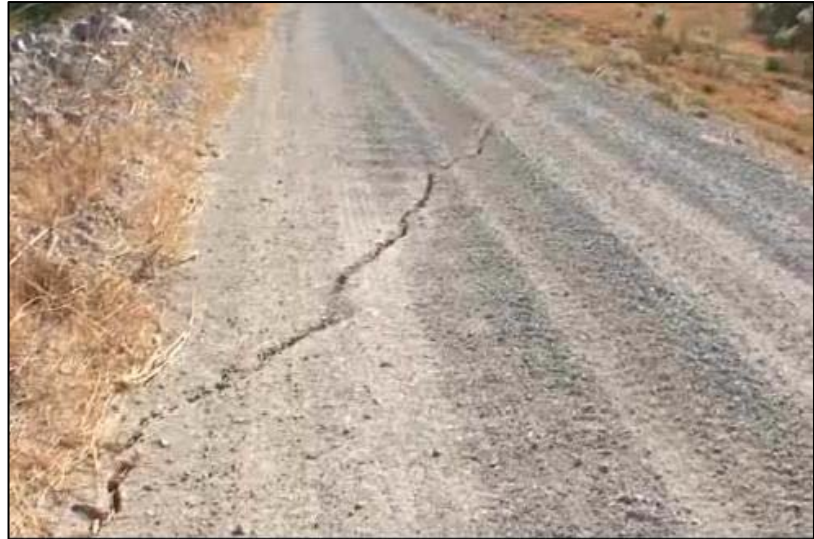
Figure 11-2: RD 2059 Levee Crack
