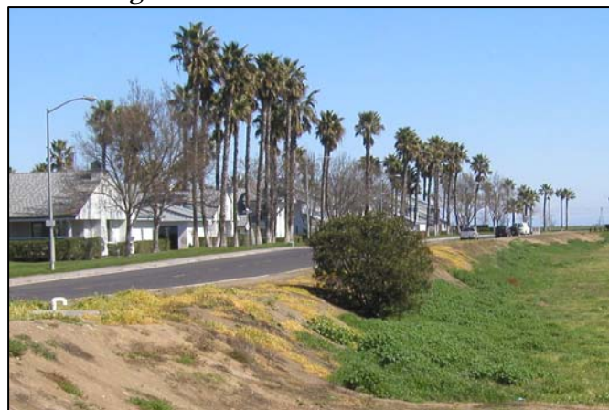
Figure 6-3: RD 800 FEMA Urban Levee
